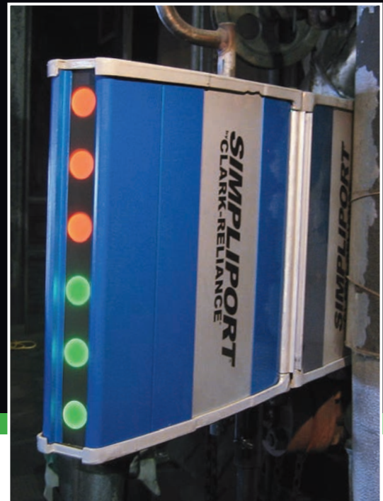
Red indicates steam, green indicates water level in boiler.
